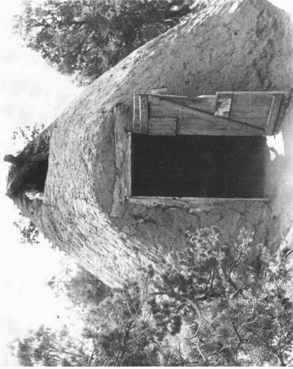
Navajo 'forked stick' hogan . A smoke hole above the fireplace is partially protected against rain. The entrance faces east. Near Betatakin, Arizona, USA.
